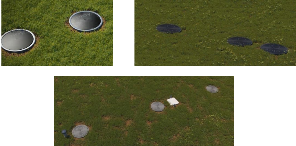
Fig-27: Completing the venting system of a single, of a two or of a three-tank Oxyfix® C-90 unit.
