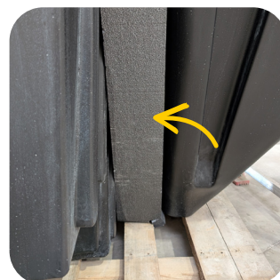
Polystyrene wedge to be kept in place during in- stallation
